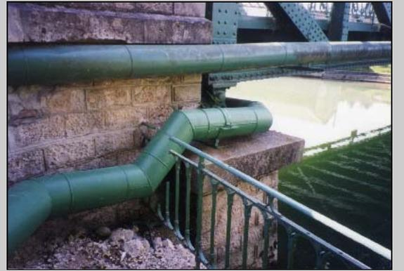
Vacuum sewer attached to the bridge abutment
